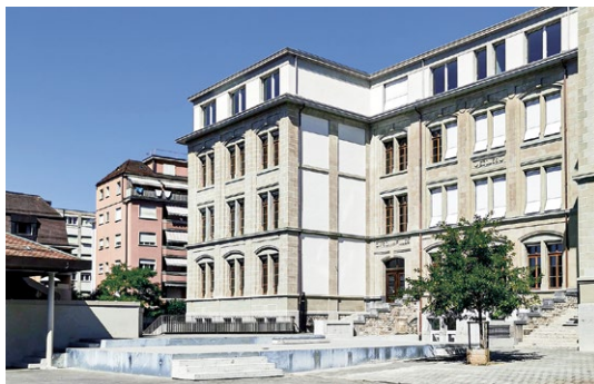
© Amsler Dom architectes
